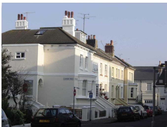
General view looking west of the houses on York Road, at the junction with Cannon Road an identified Area of High Townscape Value
